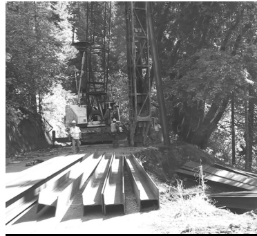
August 27. Pilings staged for retaining wall
