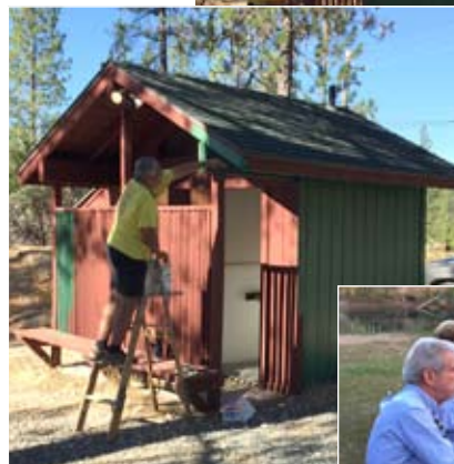
Board Members repainting the bathrooms at Lost Mine Lake
