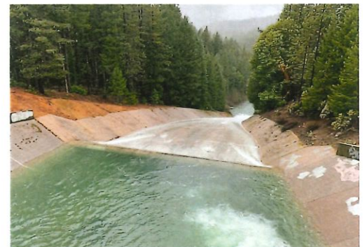
Scotts Flat Dam spillway
