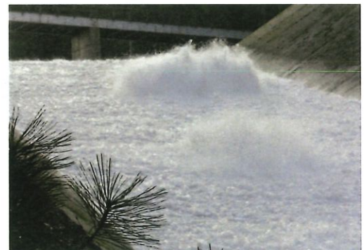
Flow disturbance caused by spalled concrete.
